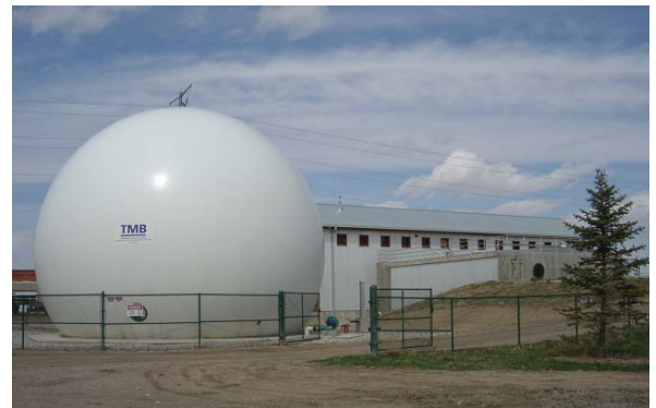
New Belgium Brewery's 225,000 gallons/day process water treatment plant with anaerobic and aerobic digestion
